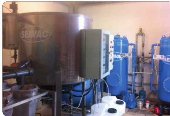
0,5-4 m3/h chemical-physical or filtration for carenage water and rain water treatment.
